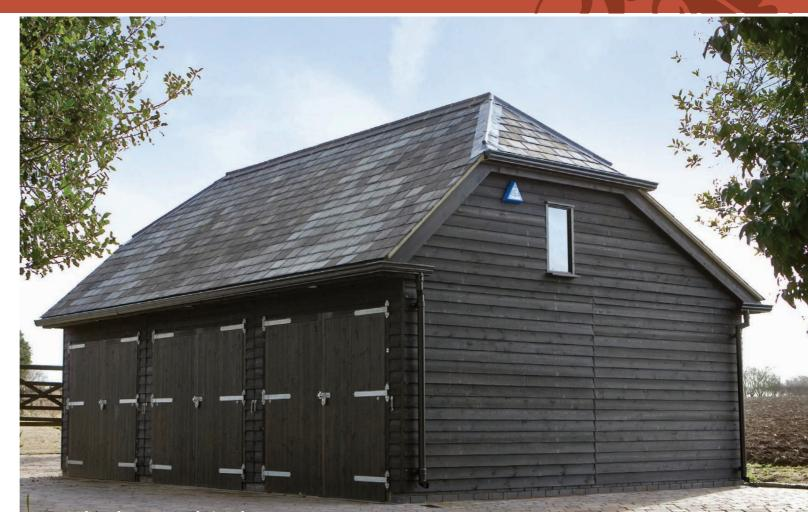
A three bay garage designed to comply with local authority planning restrictions. Dark stained, feather edged cladding with a natural slate roof.
