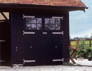
A two bay carport with secure garage area, dark stained timber cladding and a clay tile roof with Dutch hips.
